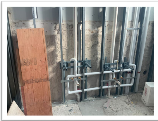
In-wall and MEP rough-ins in the gym bathrooms.
