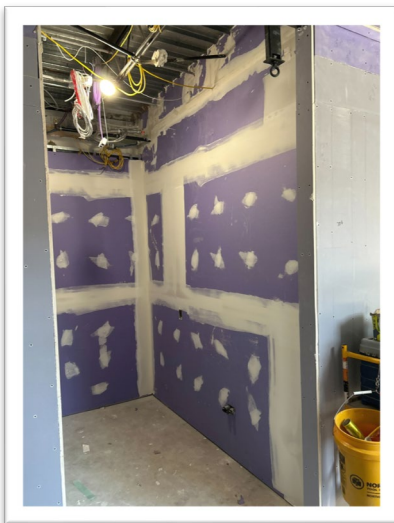
Drywall installation in the gym bathrooms.
